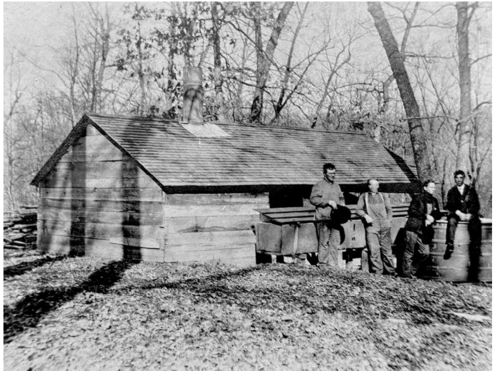
Figure 1 Open sided sugarhouse from the 1880s and 1890s built to cover a large flat pan at the Wolsfeld sugarbush. Photo courtesy of the Western Hennepin County Pioneer Association.
