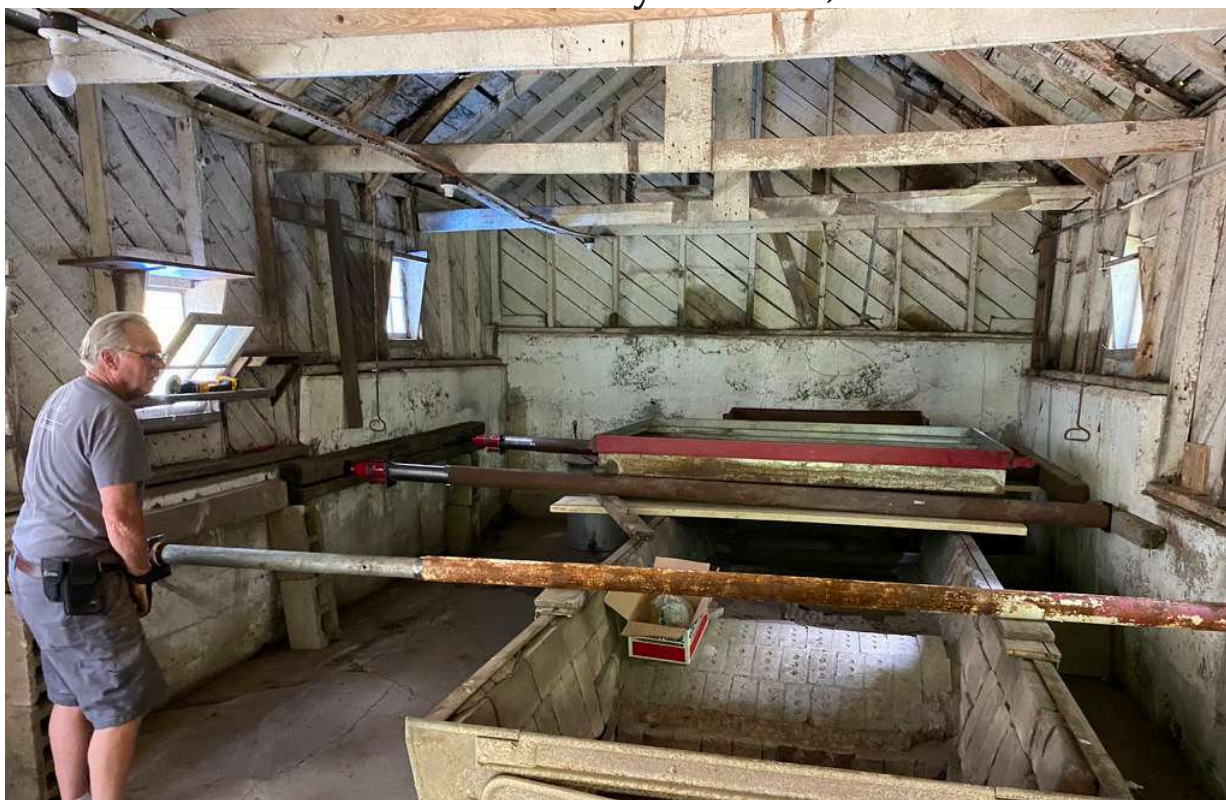
Interior wall stabilization efforts in sugar house during restoration at Green's Maplewood Farm (Image Courtesy of Green Family archives).
