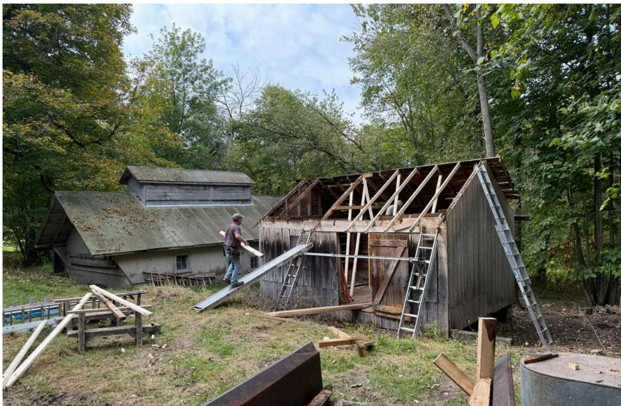
Restoration work on the cook shanty with the sugar house in background at Green's Maplewood Farm (Image Courtesy of Green Family archives).
