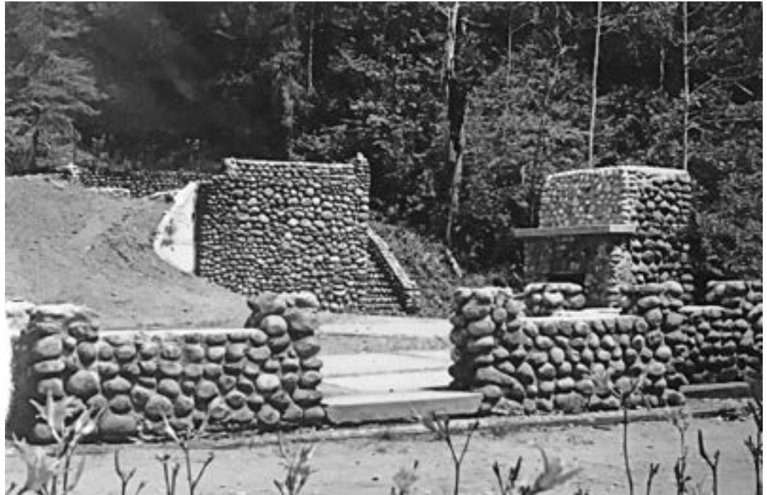
Figure 22. Remains of stone walls and foundation of the lodge at Hitchins Park near Upper Dam following removal of the structure by the Department of Environmental Conservation, circa 2000. Courtesy of Mike Romeo.
