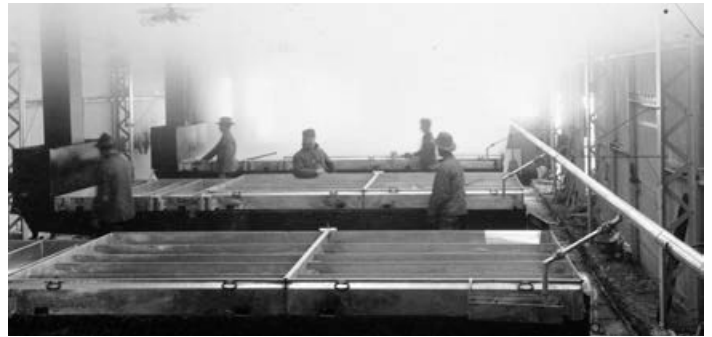
Figure 15. Interior Maple Valley sugar house with a series of enormous Champion Brand maple sap evaporators manufactured by the G.H. Grimm Company. Shows steel building walls and pipe delivery of sap. Courtesy of Library of Congress.
