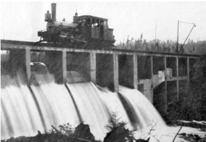
Figure 23. Lower Dam shortly after completion looking west from below the dam and showing locomotive on rail atop dam. Image taken from Ambursen Hydraulic Company Album for 1906.
