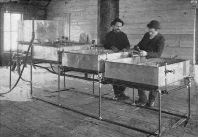
Figure 3. Two men, possibly James Hill and John Rivet, standing alongside a model of steam heated evaporating pan for making maple syrup, identical to an evaporator in patents sponsored by A.A. Low. Image taken from Fox and Hubbard booklet, The Maple Sugar Industry from 1905.
