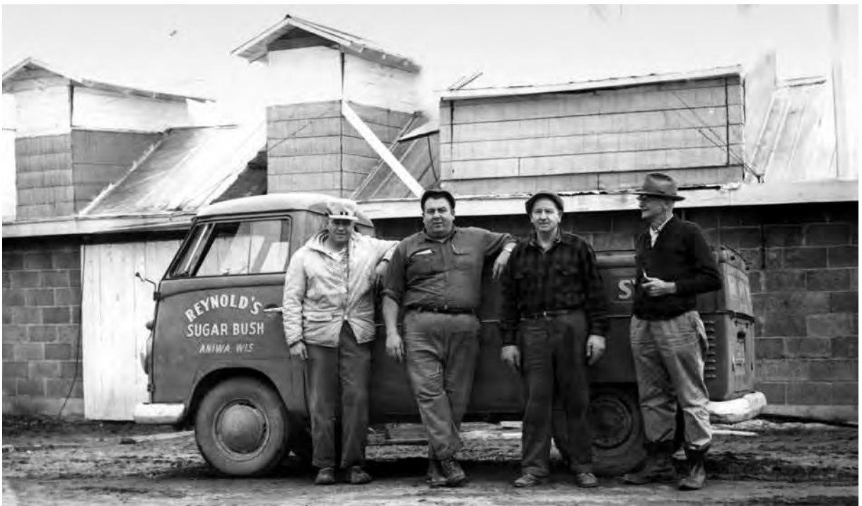
Top: Each Reynolds plant boasted two or three massive six-foot-by-eighteen-foot stainless-steel evaporation pans fueled by a series of oil-fired burners. Standing in front of one such evaporator, left to right, are Adin, Lynn, and Juan Reynolds and Bob Lamb, ca. 1960. Bottom: The fame and growing influence of the Reynolds Sugar Bush prompted a visit from Bob Lamb of Bernhards Bay, New York. Lamb was an early inventor of flexible plastic tubing used for gathering maple sap. From left to right are Lynn, Juan, and Adin Reynolds and Bob Lamb in front of the Aniwa plant, ca. 1960.
