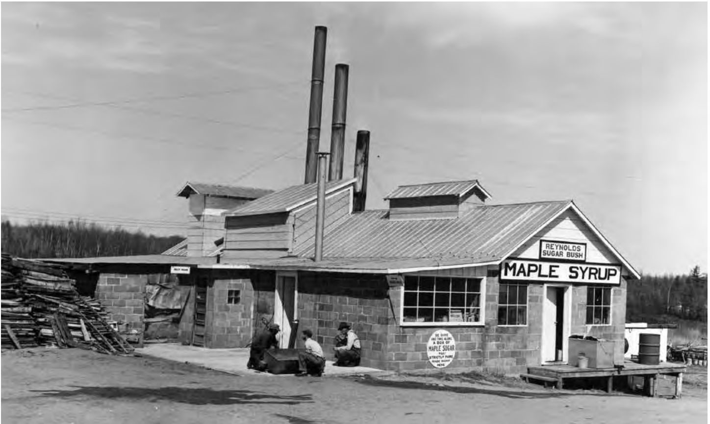
The Reynolds Sugar Bush began its life with the construction of this syrup plant in 1947. In the beginning, the plant featured two wood-fired evaporators, but rapid growth of their business led the family to expand the plant with the addition of a third evaporator and conversion of all evaporators to oil fired. Note the stacks of waste wood from the sawmill to the left.
