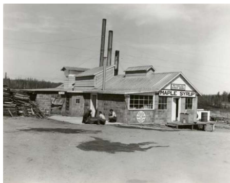
Image of the new Reynolds Sugar Bush building in 1954. Photo by Dean Tvedt. Source: University of Wisconsin-Madison archives
