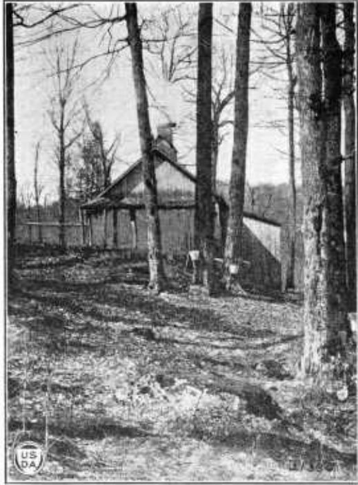
FIG. 10.—This boiling house stands on high ground, but the gathering tank may be emptied by gravity. The sides of the house are tight and a ventilator on the roof allows the steam to escape.
