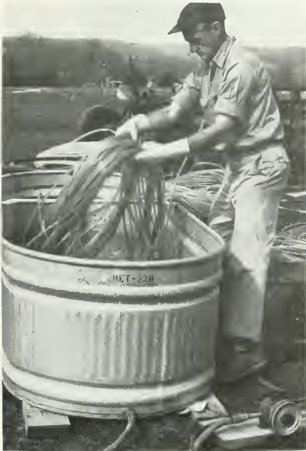
Figure 57.—Coils of lateral lines are submerged in hypochlorite solution, and all the ties are cut except those at the end of the bundle.
