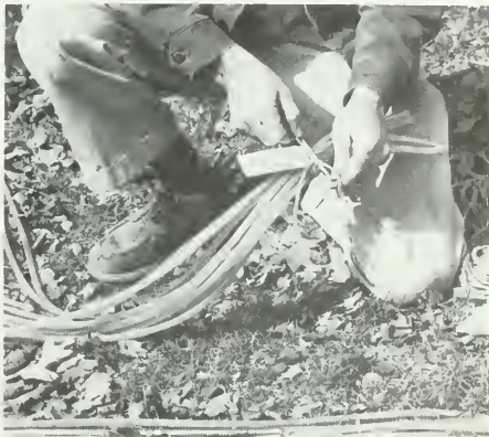
Figure 54.—Tying and labeling bundles of lateral lines.
