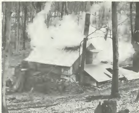
Figure 68.—Evaporator house located in center of sugar grove. Without a covered evaporator, steam completely fills the evaporator house. This is unfavorable for sanitary conditions.
