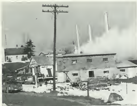
Figure 125.—A large central evaporator plant located at Anawa, Wis. Some plants are large enough to make 20 or more gallons of sirup per hour.
