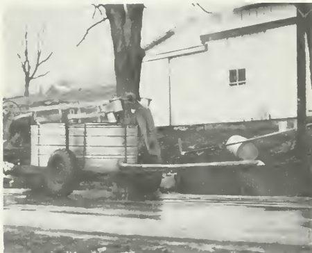
Figure 65. —This receiving tank is mounted at the roadside. Sap is pumped from it to the evaporator storage tank.
