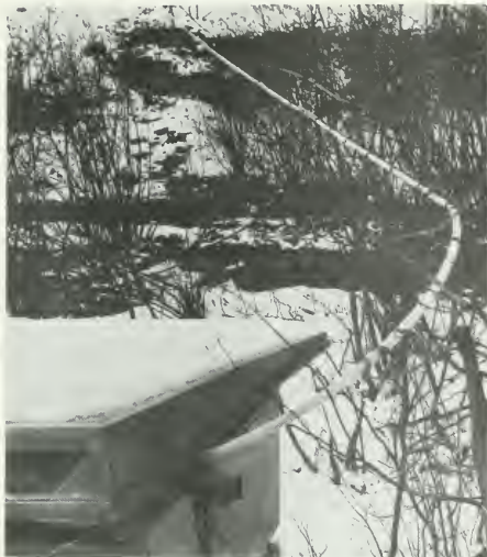
Figure 47.—Main line to roadside tank for pickup.
