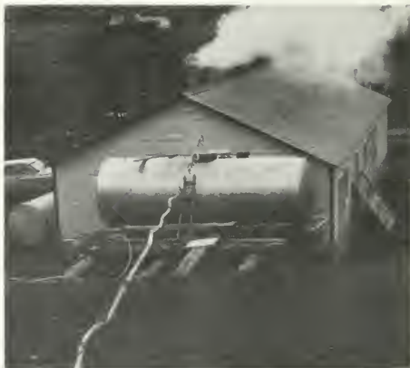
Figure 46.—Main lines transport sap to storage tank at the evaporator house.
