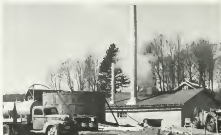
Figure 124.—This central evaporator plant at Ogema, Wis., has one evaporator.
