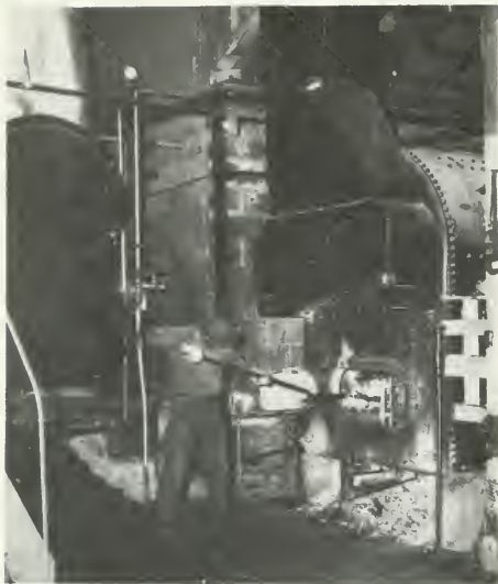
Figure 84.—High-pressure steam boilers are economical when low-priced fuel is available. Approximately 20 gallons of finished sirup per hour can be made in the two 100-h.p. boilers shown.
