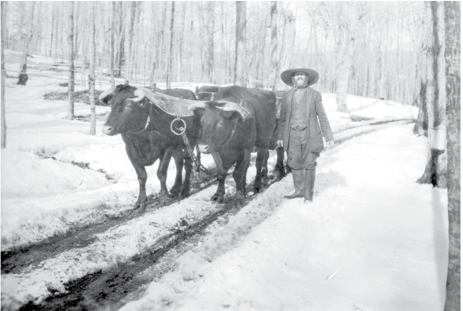
Albert Leland leading a team of oxen pulling gathering tank on a road through the sugarbush where metal pipeline is being used. Photo from the Tom Olson Collection
